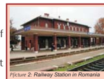
Picture 2: Railway Station in Romania
